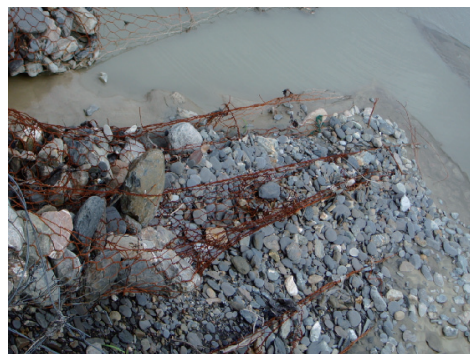
(f) 蛇籠護岸工程破壞案例 6 (f) Roll gabion revetment failure case No.6
